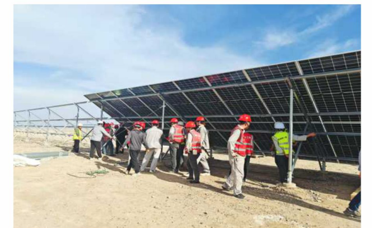
PV Support Structures for Guangdong Energy Group Shache County 2000 MW PV-Storage Integrated Project (550 MW) EPC
